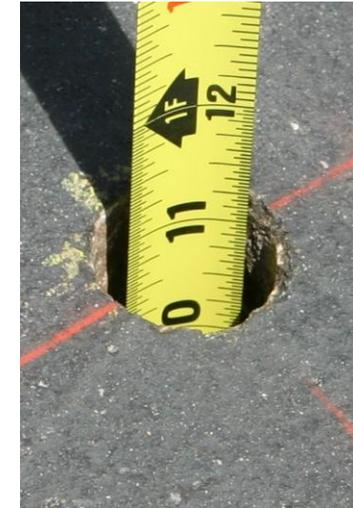
7. Saw cut the four legs of the loop to a minimum depth of 1.5 inches with a 1/4 inch saw blade.
